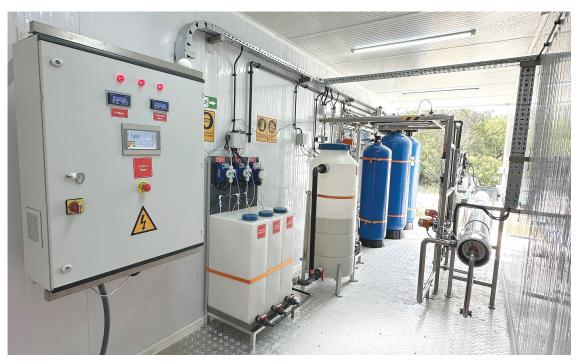
Miranda's RO / Cell containerized water treatment plants are designed to treat water 40 - 240 m3/day of either brackish, contaminated or seawater with an output of potable water.
